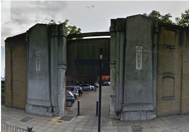
Image showing Grade II listed Entrance Gateway
